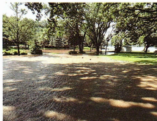
Figure 3 – Flooding Downstream of USH 45 Culvert
